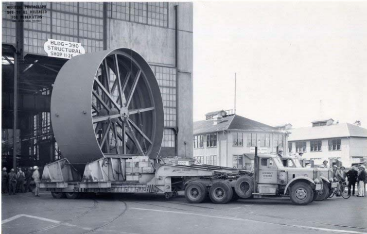
First Hull Section being moved to Building Ways
