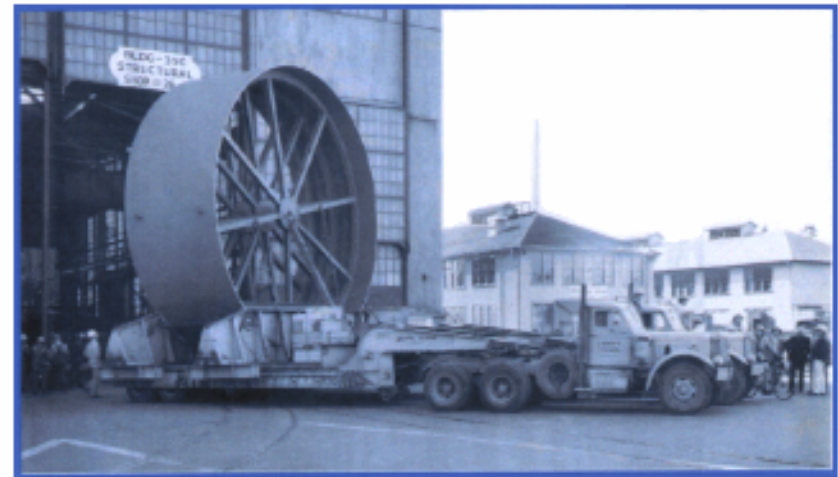
First Hull Section being moved to Building Ways 14 February 1956
